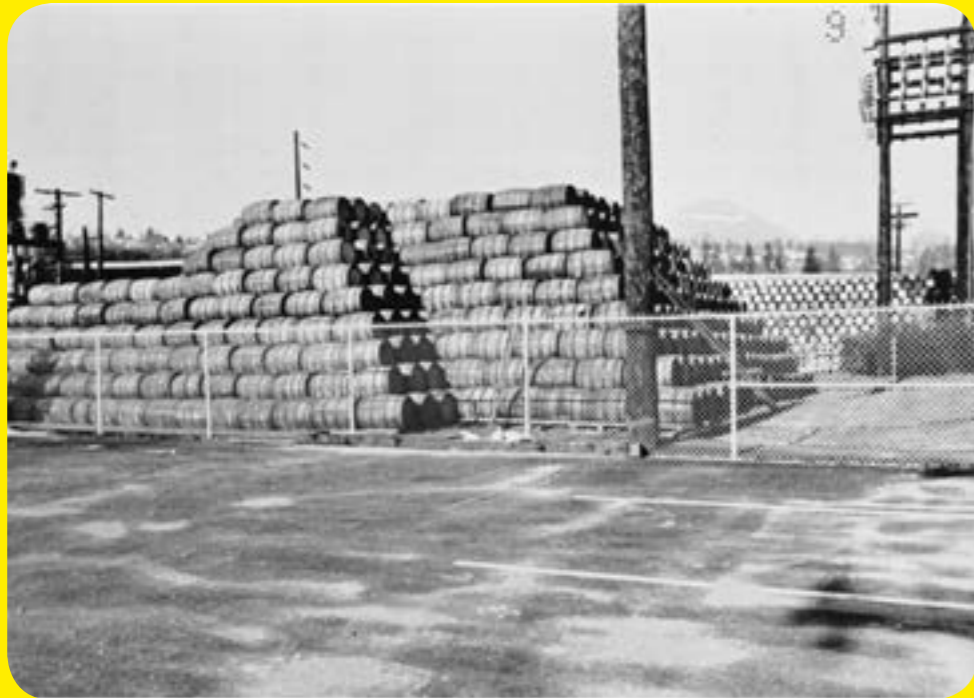
9. Canadian Park and Tilford Distilleries Limited, Corner of Brooksband and Main, North Vancouver, B.C.
